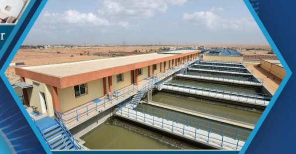
10 th of Ramadan Potable Water Plant
