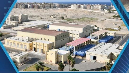
El Yosr Seawater Desalination Plant - Hurghada
