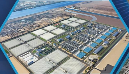
Bahr El Baqar Treatment Plant
