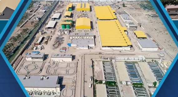
Basra Desalination Plant - Iraq
