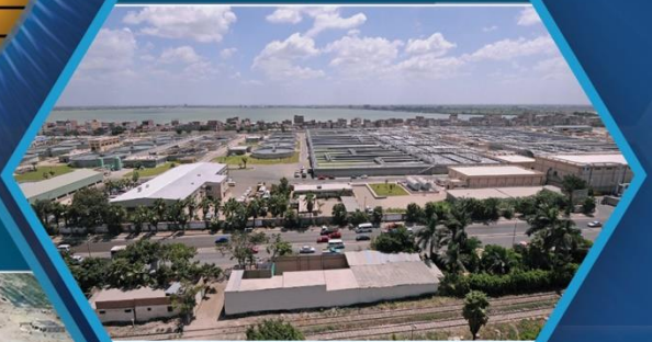
Eastern Wastewater Treatment Plant - Alexandria
